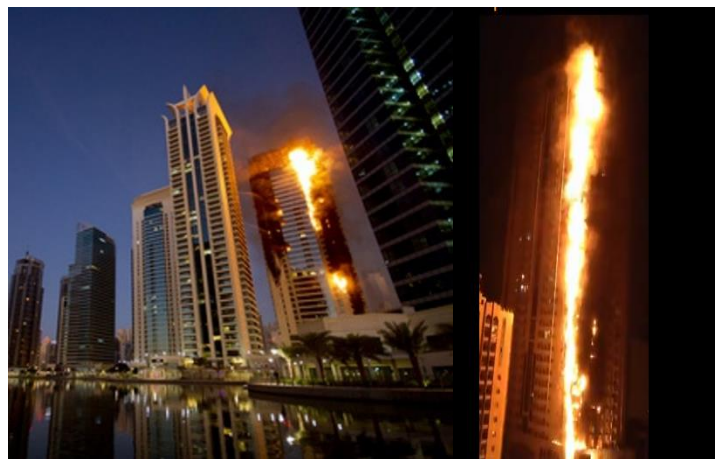
Fig. 6 34-storey building fire, Dubai, the United Arab Emirates
