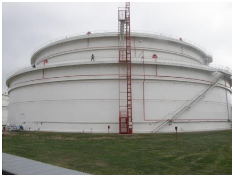
Figure 3 Storage tank with capacity of 70 000 m 3
