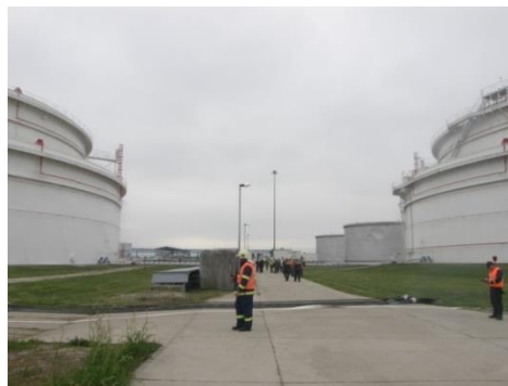
Figure 1 Crude oil pump station in Tupa
