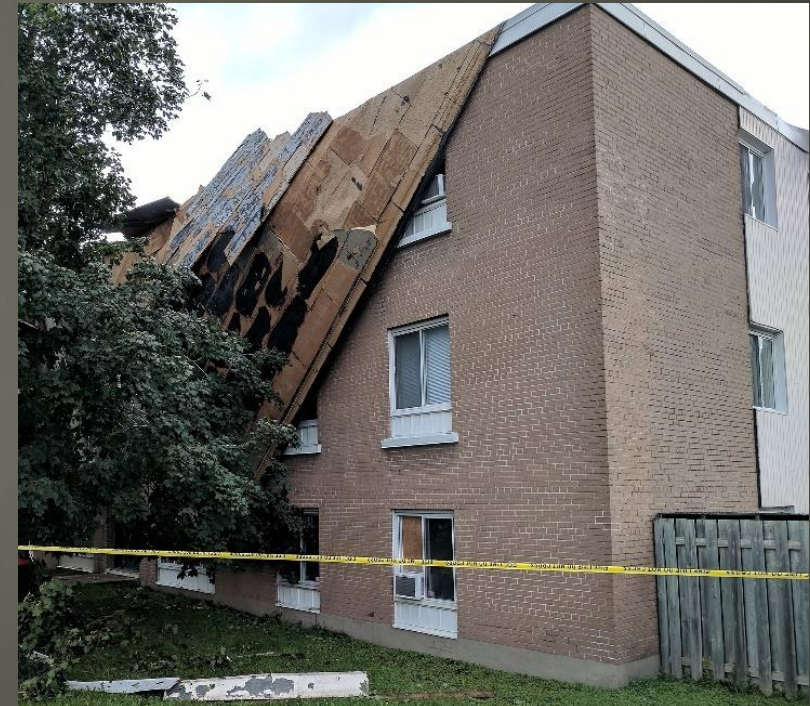
Roof delamination from wind effects
