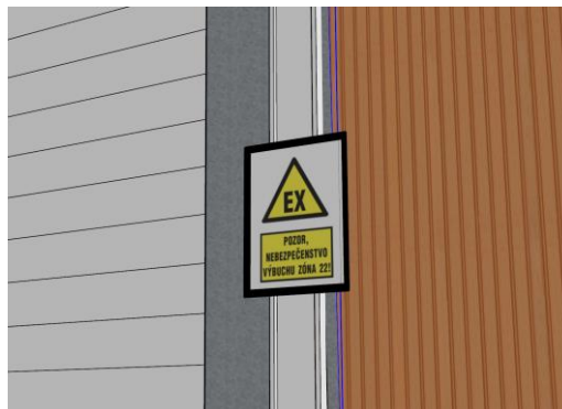
Fig. 17 Marking of entry into an explosive atmosphere
