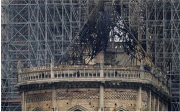
Fig 7. Wrenched scaffolding
