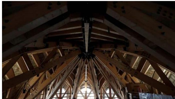
Fig 13. Wooden beams supporting vault
