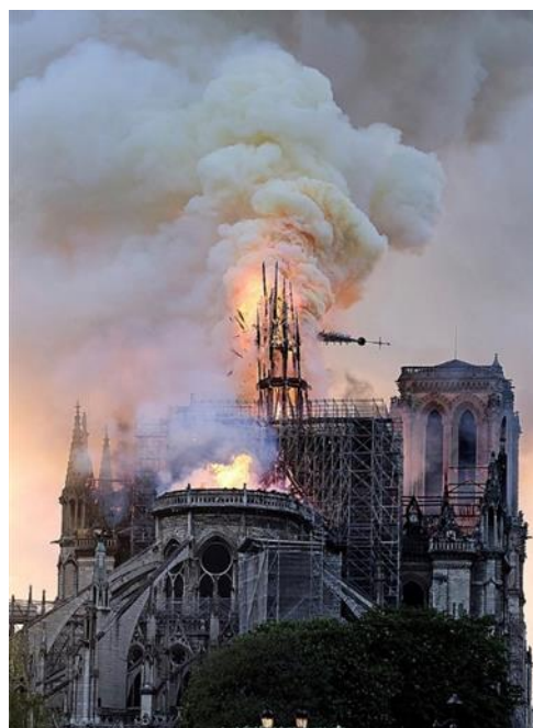
Fig 4. Collapse of the Sanctuary tower
