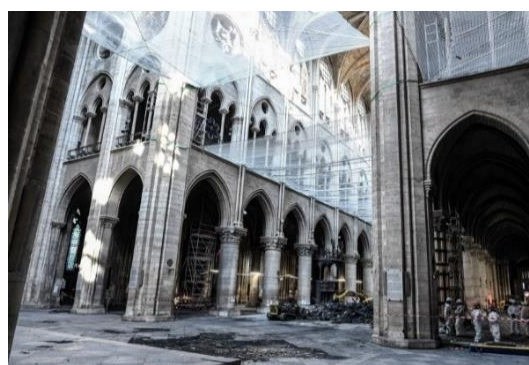
Fig 15. Reconstruction work indoors
