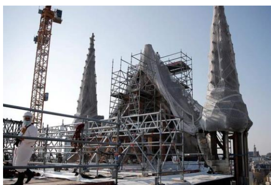
Fig 14. Current reconstruction work
