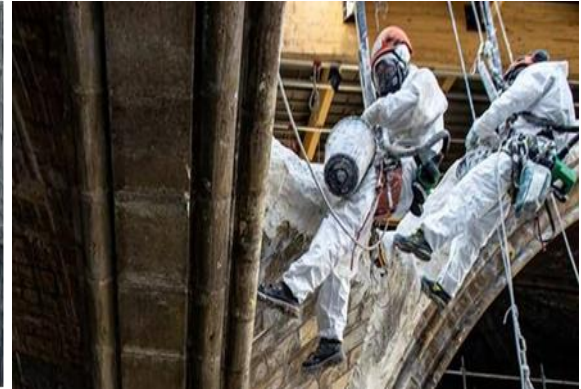
Fig 8. Rappelling workers in protective suits
