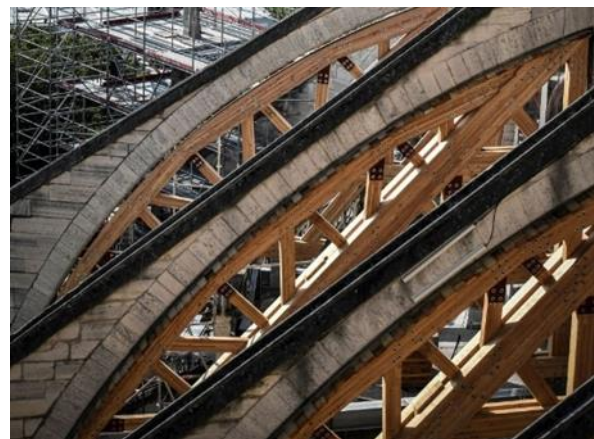
Fig 6. Wooden support vaults
