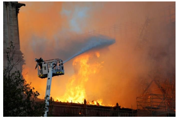
Fig 3. Fire extinguishing from platform
