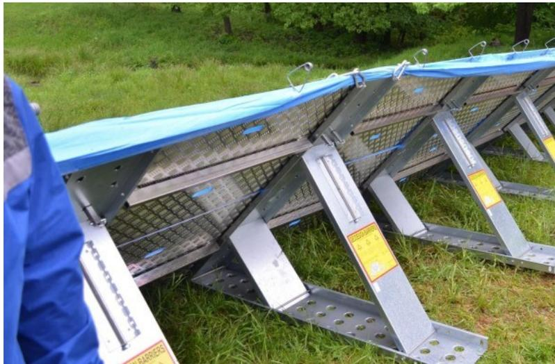
*Figure 7.3 Mobile flood barriers - part of the state material reserves*
