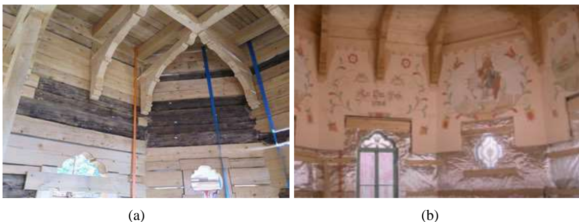
Fig. 2 (a) Log cabin wall with built-in original beams (Novák, 2018); (b) Paintings and frescoes in the new dining room, the vapour barrier is also visible in the lower part (Masák & Partner s.r.o., 2021).
