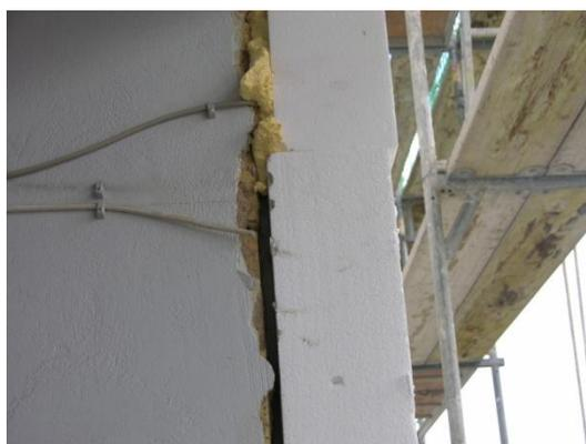
**Figure 3 Fire loads behind the insulation and bonding of polystyrene plates**
