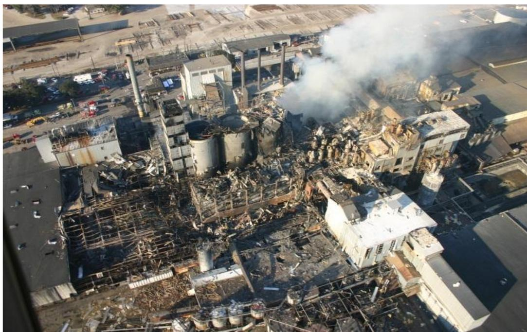
**Figure 11 “Imperial Sugar Company” in the USA after an explosion of combustible sugar dust in 2008, causing 14 deaths and injuring 38 others [3]**
