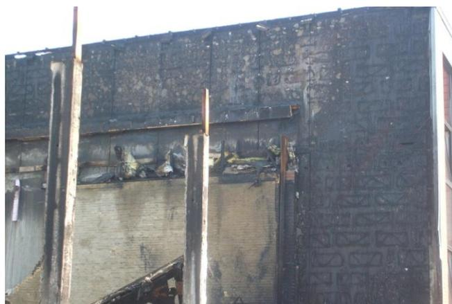
**Figure 5 This facade with EIFS burned down to the complete surprise of the fire fighters in 30 seconds**
