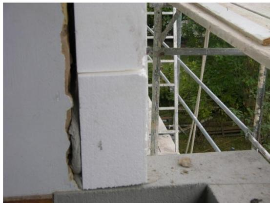
**Figure 4** The picture shows a typical installation of the defective EIFS without compliance
