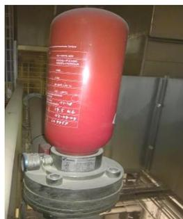
**Photo 4. Fire fighting system on the de-dusting channel**
