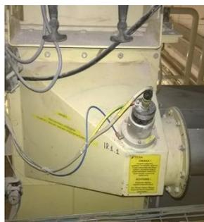
**Photo 5. Flame photosensor in the de-dusting channel**
