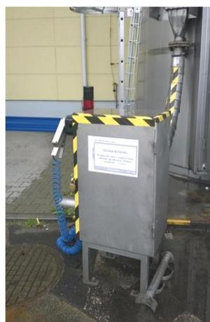
Photo 2. Cabinet with connection stub and ground monitoring system
